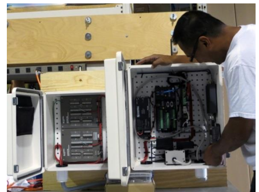
Preparing datalogger for installation
