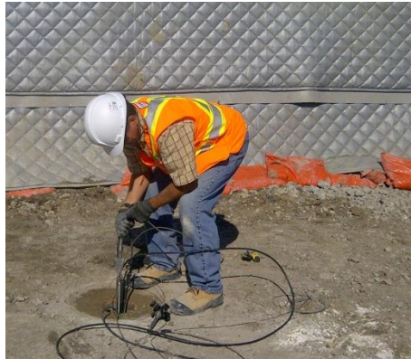
Installation of in-place inclinometer for automated monitoring
