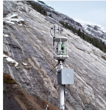
Total Station installed within the BC interior
