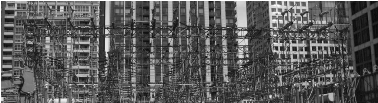
Figure 3 The hydro towers that were monitored (Monir Precision Monitoring, 2008)
