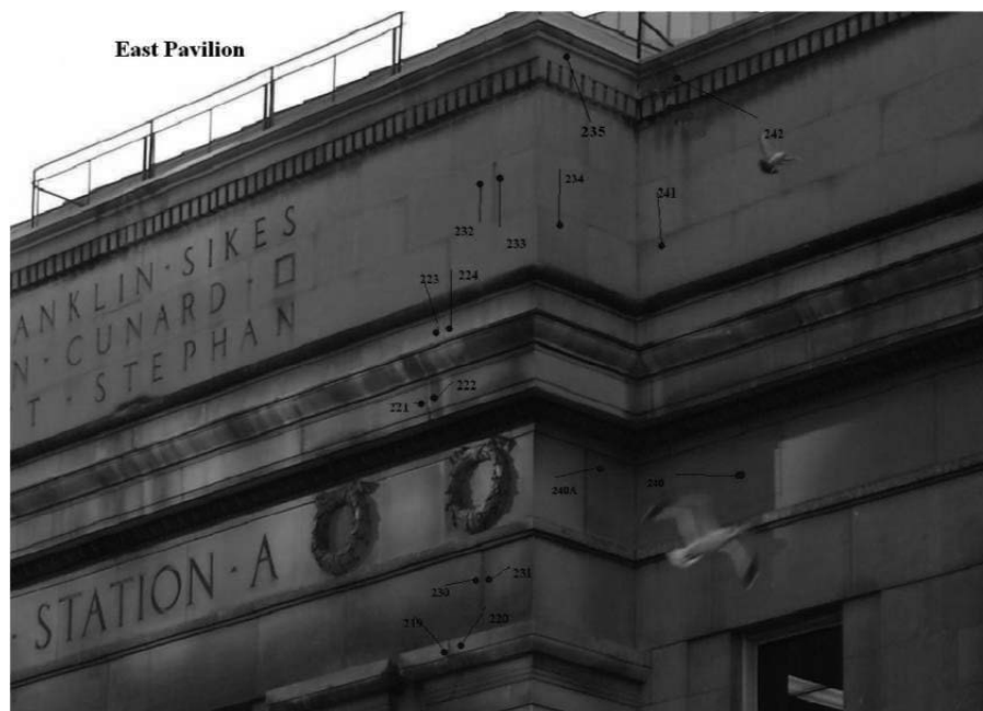
Figure 7 Monitoring points on the Head-House (Monir Precision Monitoring, February 2011)
